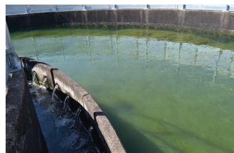
Accelerator with sludge blanket
